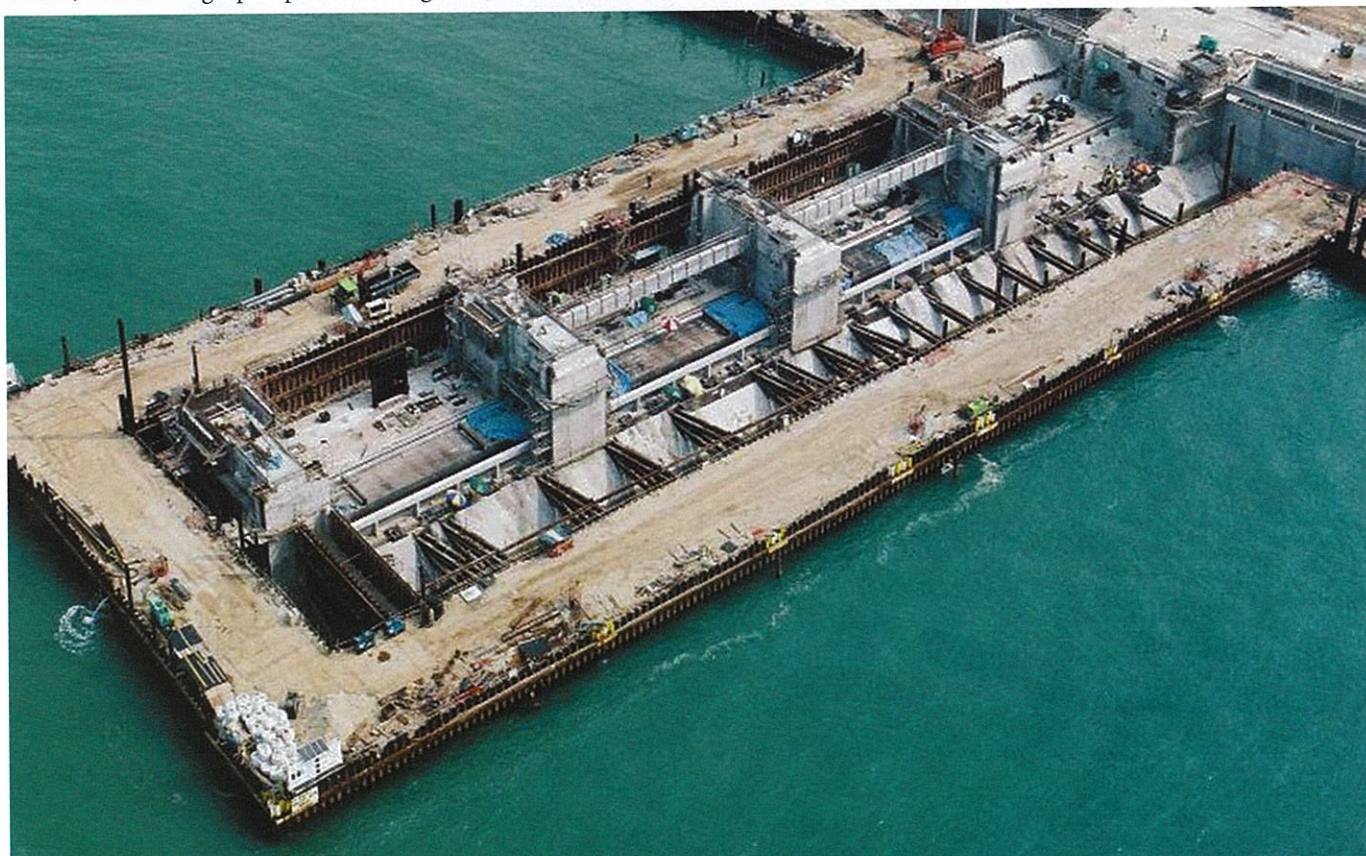
Aerial view of the double wall marine cofferdam.
