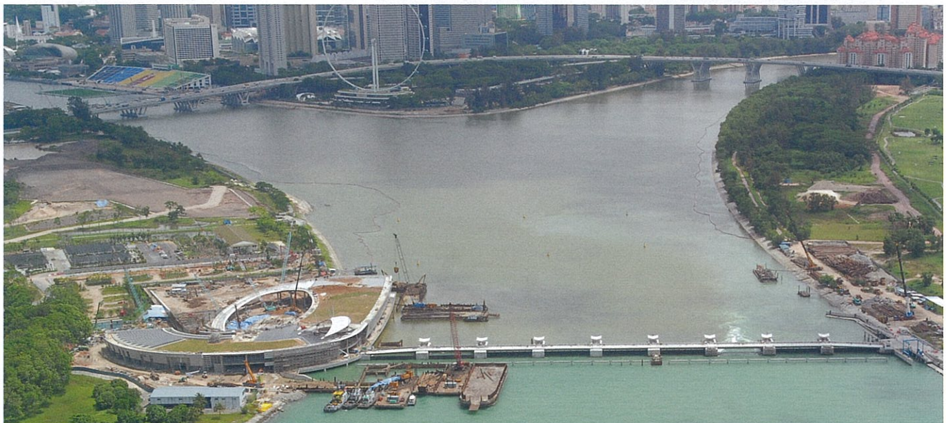
Aerial view of Marina Barrage during the construction stage.
