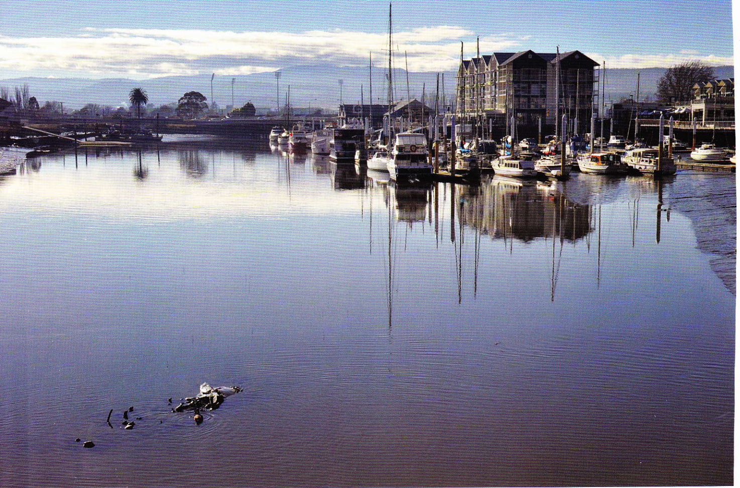
A silt-choked Seaport Marina on the North Esk 2012. For the past two years the silt has been “prop-washed” into the channel using a powerful fishing vessel
